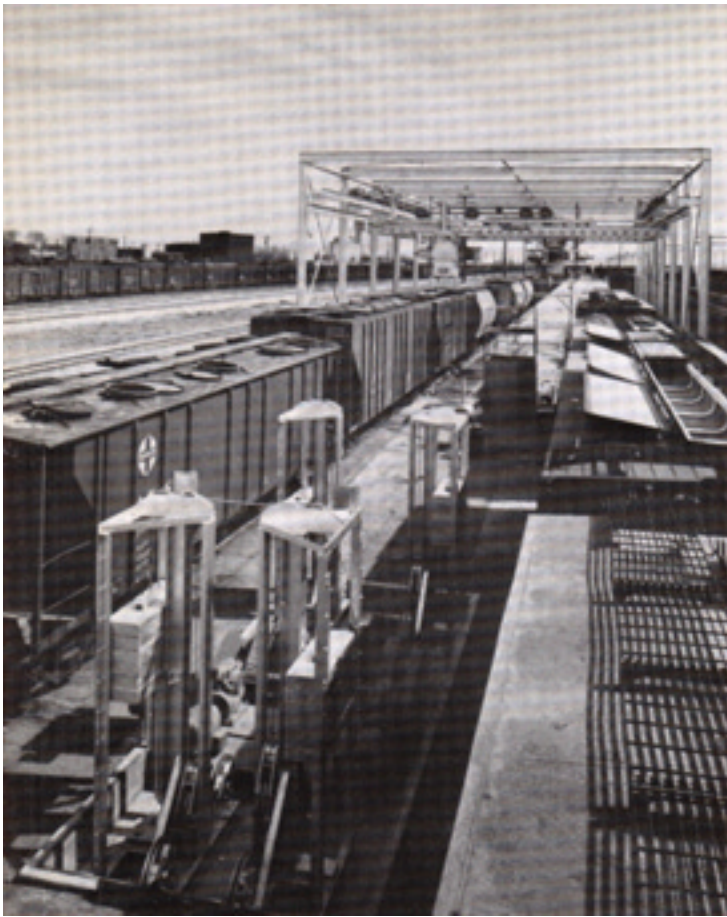
View looking in direction of car progression shows double drum continuous wire rope pullers and counterweight towers of ROBOT car progression system in foreground.
