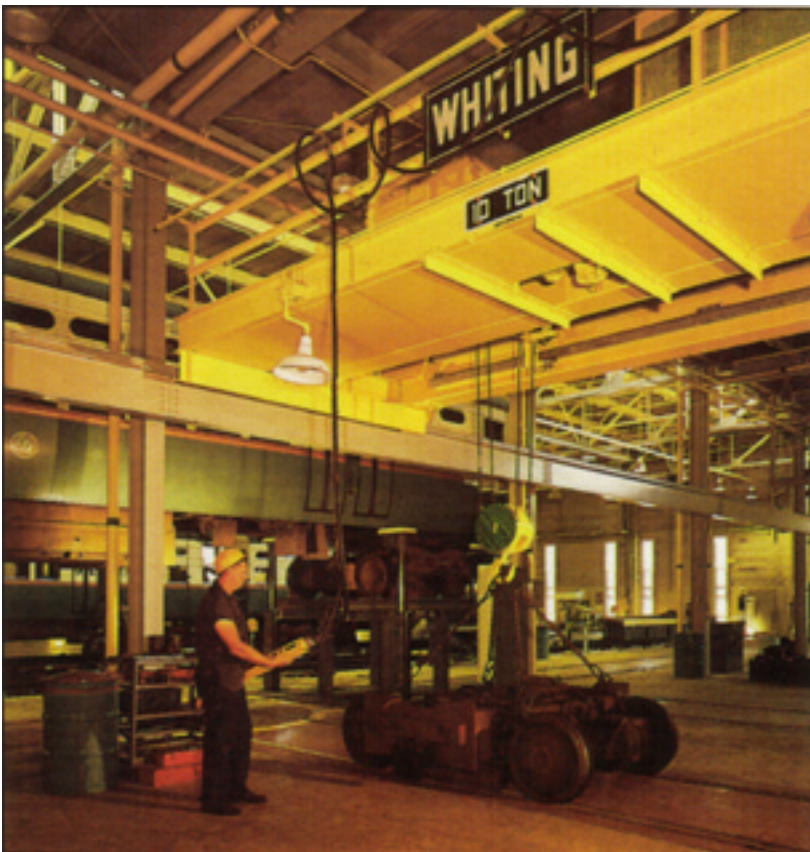
Overhead cranes for transit maintenance and repair shops
