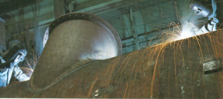
Shop view of Swenson vessel in fabrication
