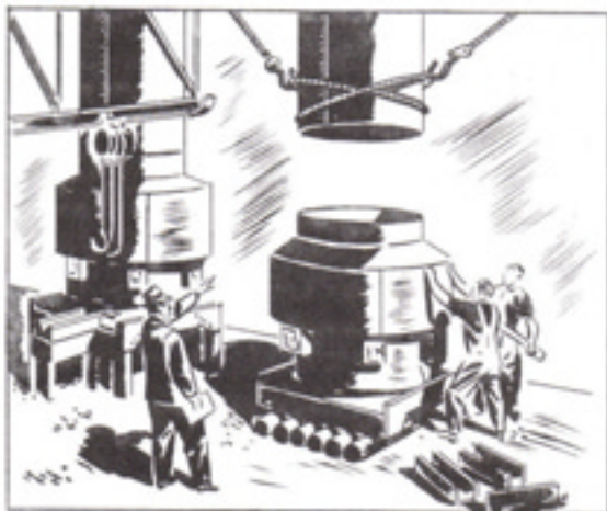
Fig. 2. Erecting a Whiting Cupola
